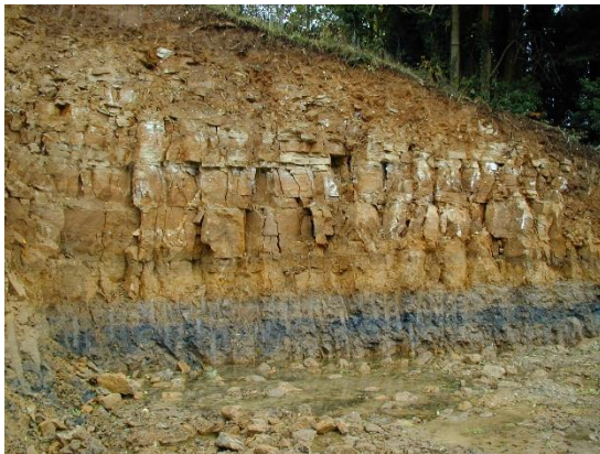
Groundwater emerges at the transition from marl, a rock with low water permeability, to sandstone, a rock with very good permeability and many joints (Photo: excavation at a construction site in the Natur- & UNESCO Global Geopark, SGL).
